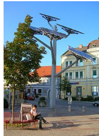
Photovoltaic system 'tree' in Styria, Austria
